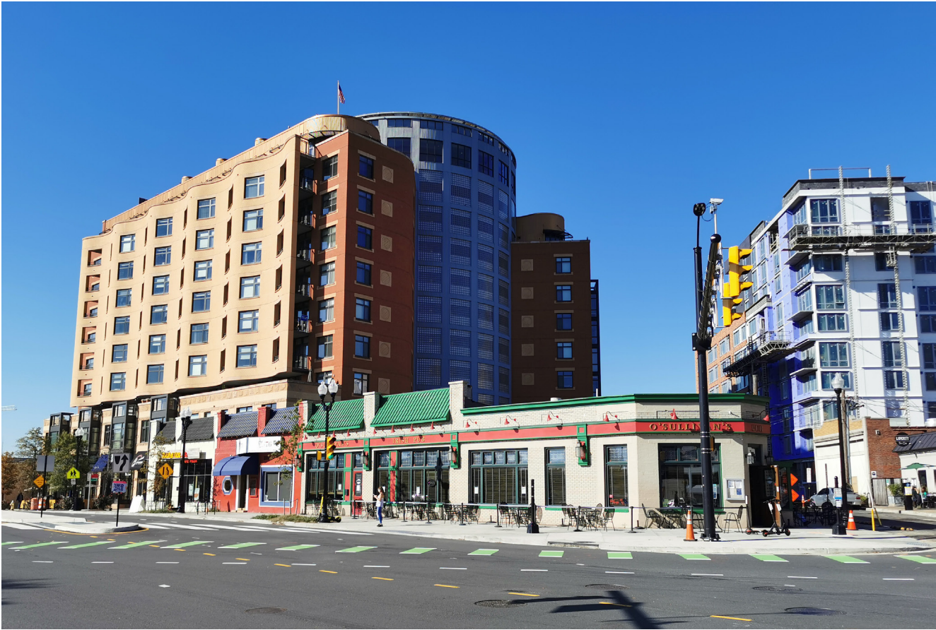
LOOKING NORTH WEST - WASHINGTON BLVD AND WILSON BLVD (O'SULLIVAN'S IRISH PUB)
