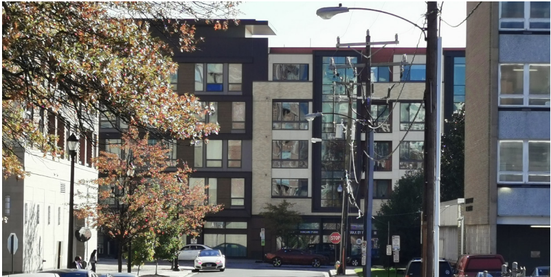
LOOKING SOUTH - N. IRVING ST.
