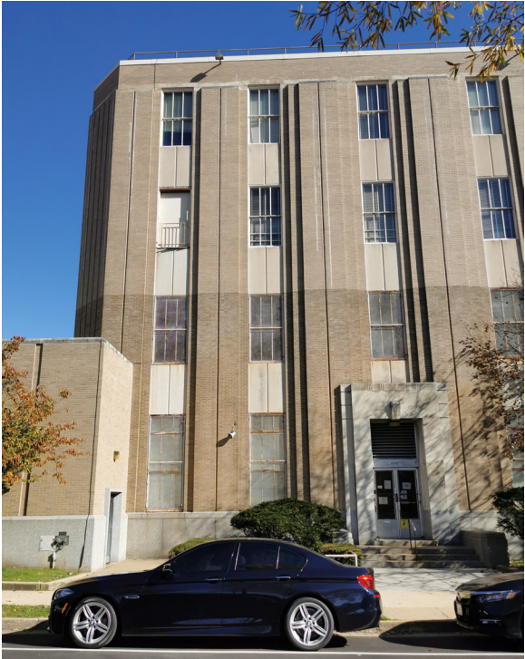
LOOKING EAST - N IRVING ST (VERIZON)
