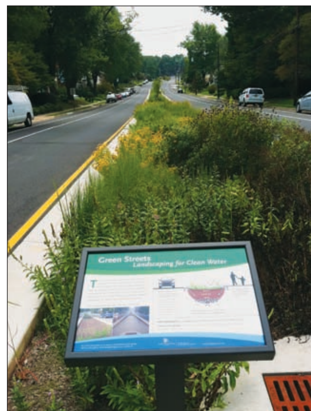
This Green Street facility on Patrick Henry Drive filters stormwater runoff before it enters Four Mile Run.
