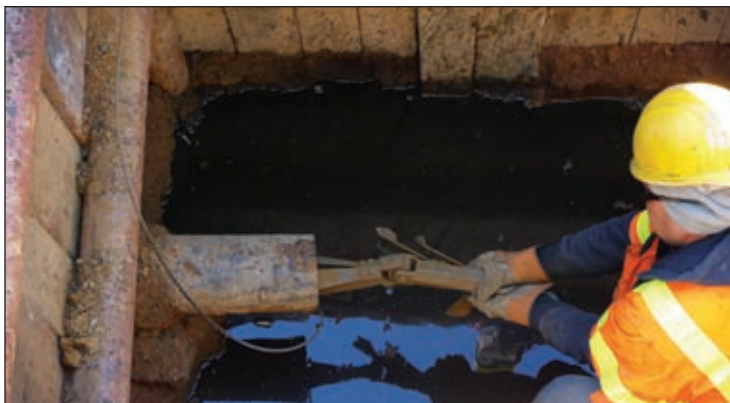
A worker in an access pit handles a mechanical scraper used for cleaning water mains.
