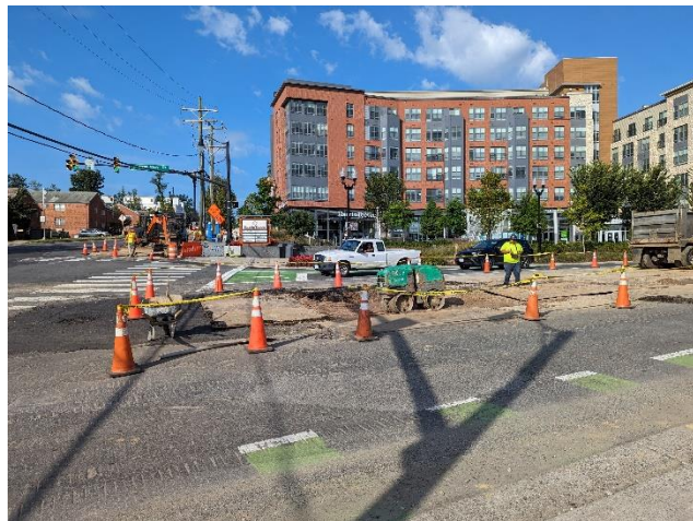
Construction site on S George Mason Dr
