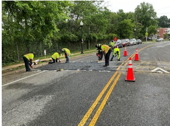
Installation of a tactical speed hump
