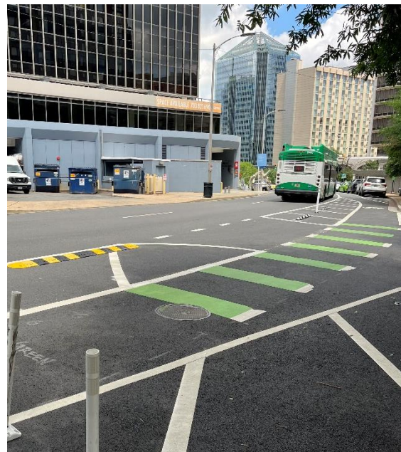
Enhanced roadway markings, flex posts, and raised speed humps installed along downhill bike lane at right turn conflict
