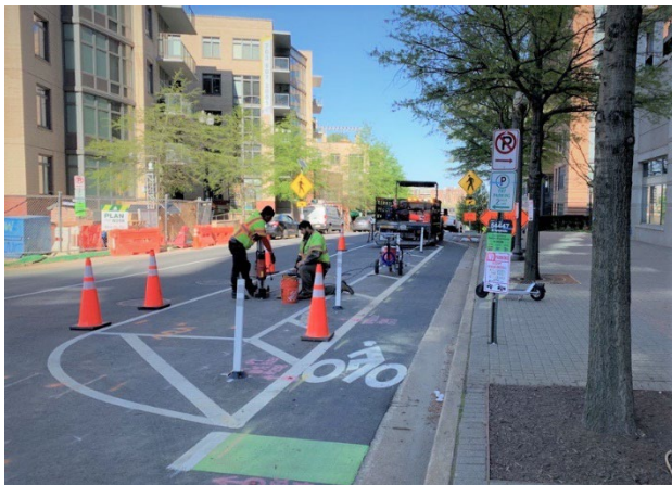
Street boring and sensor installation
