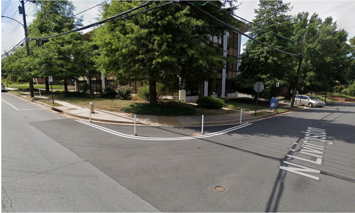
Figure 6: Existing Tactical Curb at corner of Wilson Boulevard and North Livingston Street
