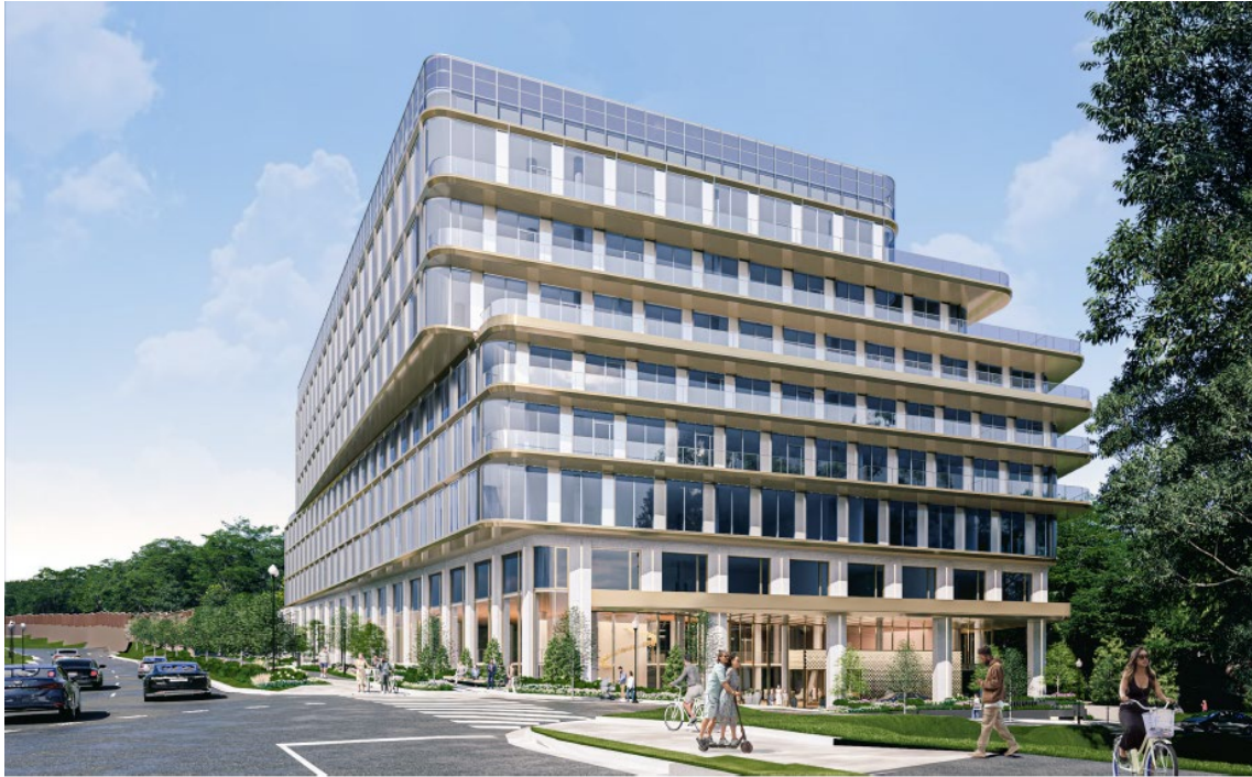
VIEW FROM LANGSTON BLVD
