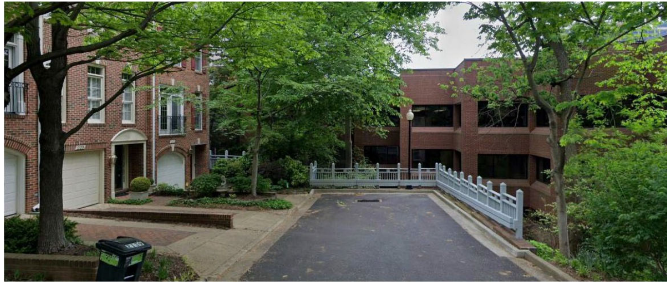
NORTH PIERCE COURT WITH EXISTING AFA BUILDING
