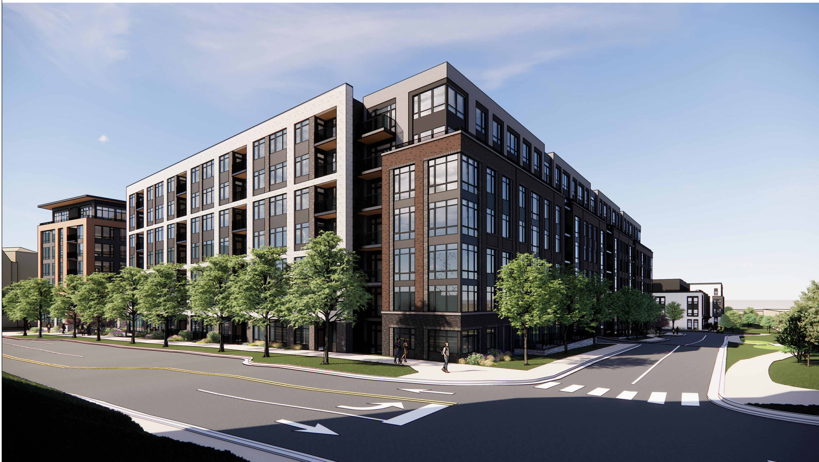
3 --- BLDG E - NORTHWEST VIEW
