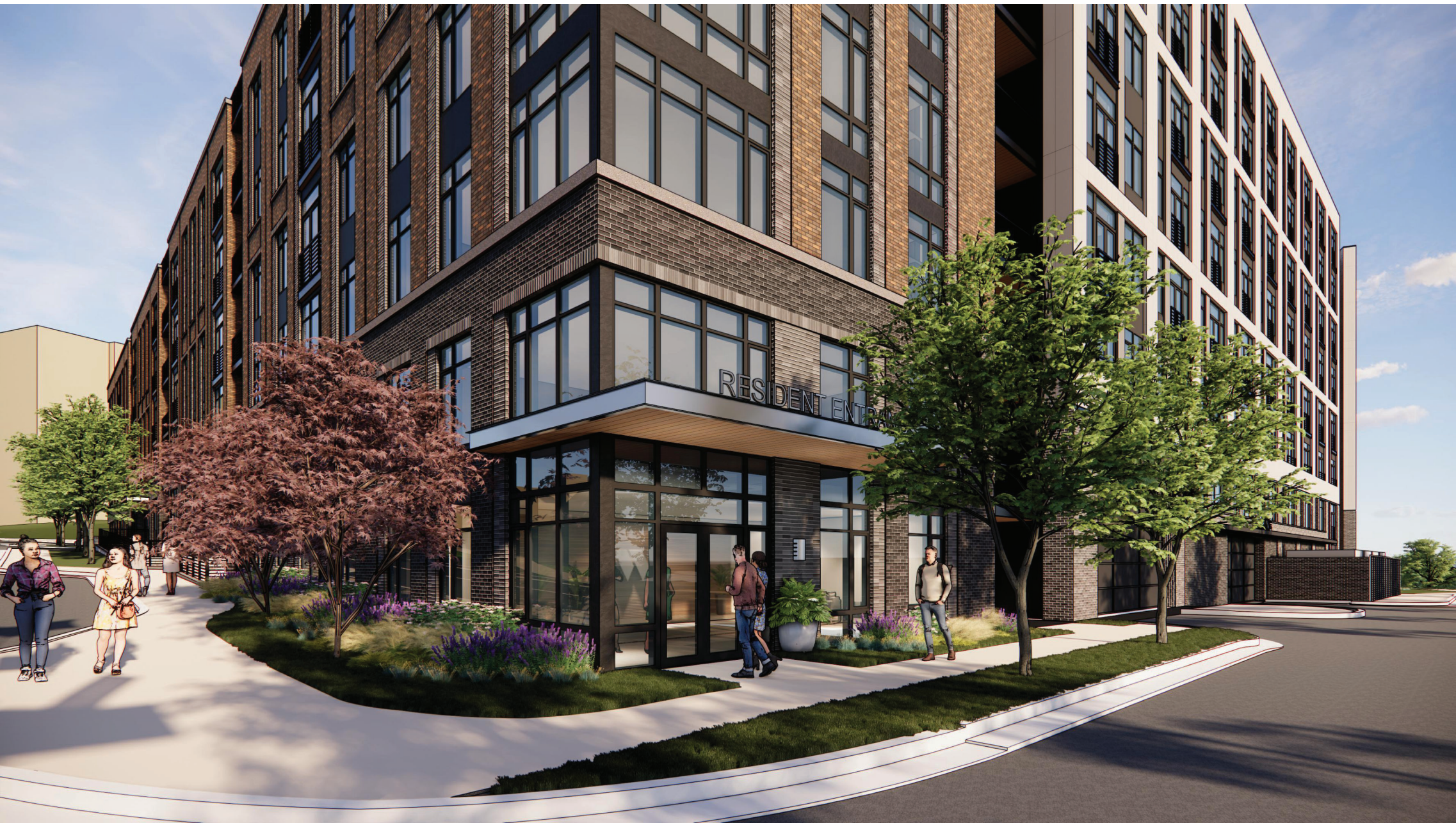
2 --- BLDG E - SECONDARY ENTRANCE OFF PRIVATE DRIVE
