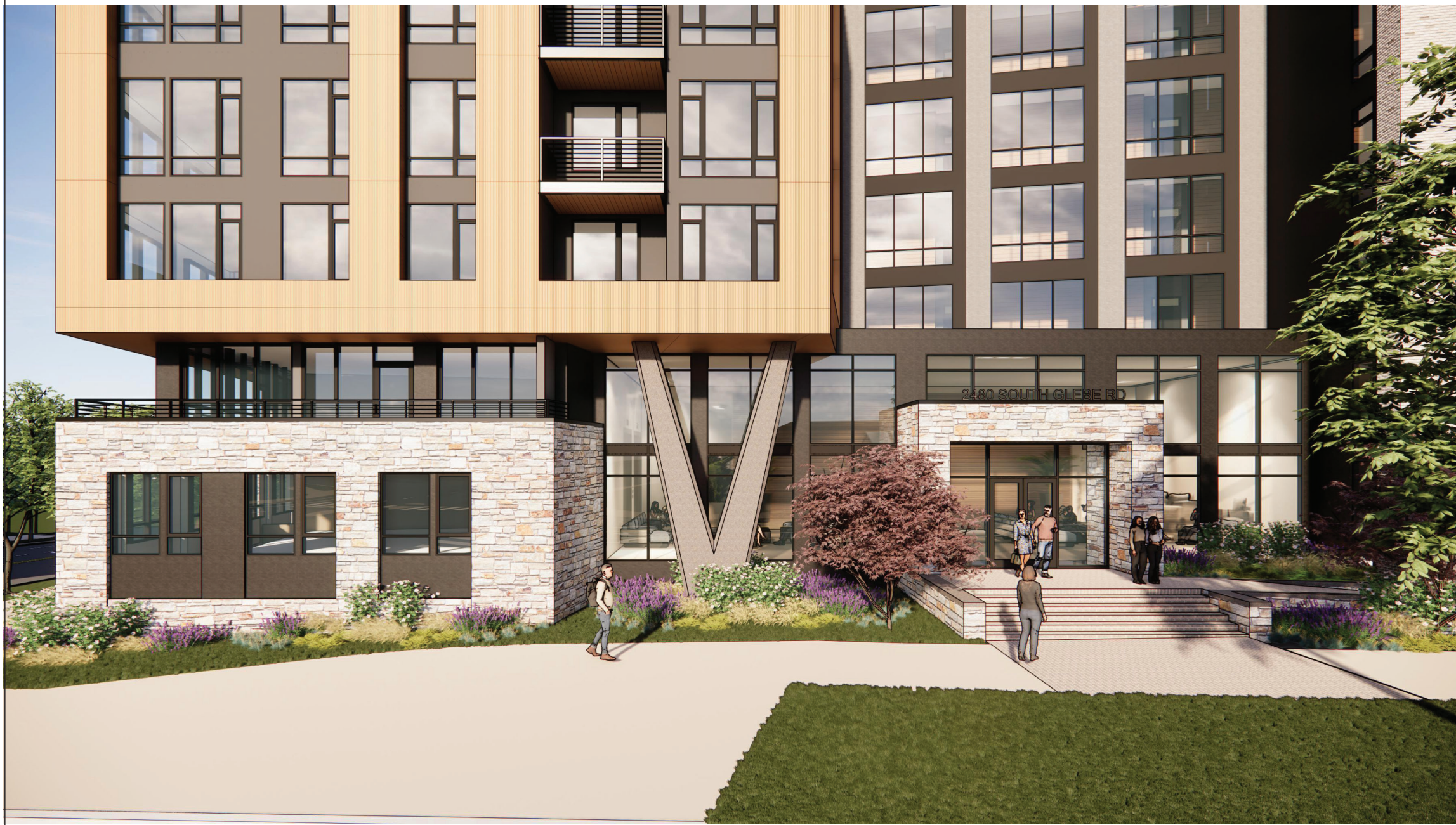
3 --- BLDG E - MAIN ENTRY CLOSEUP
