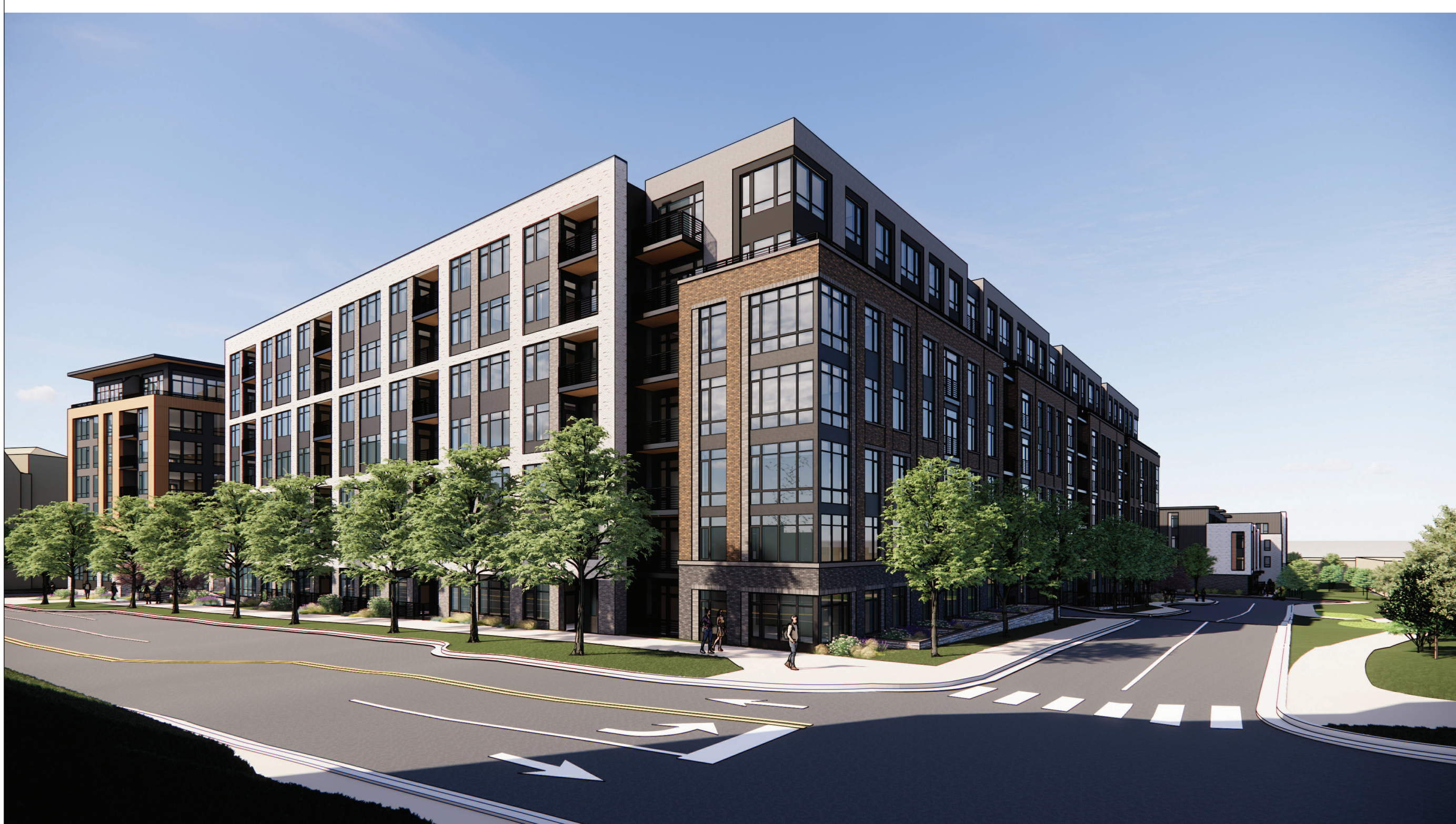
3 --- BLDG E - NORTHWEST VIEW
