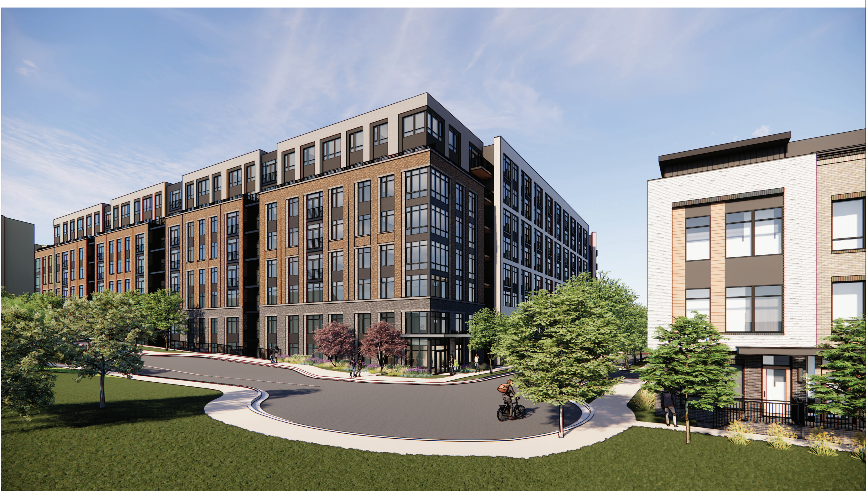
4 --- BLDG E - SOUTHWEST VIEW
