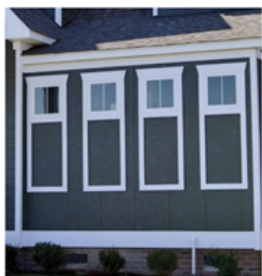
improper window framing
