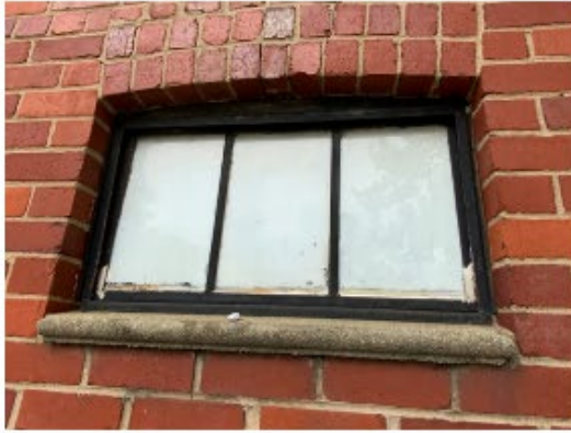
EXISTING BASEMENT WINDOW
