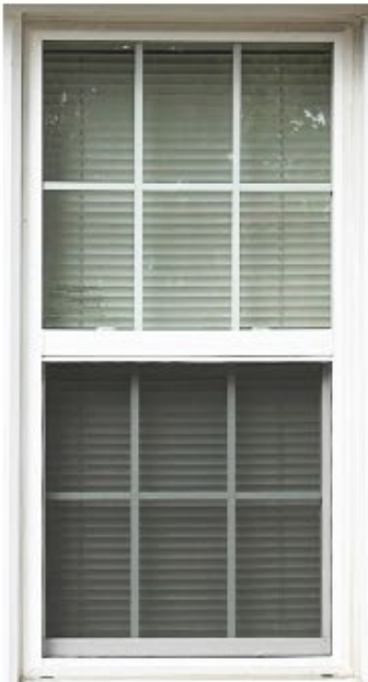
TYPICAL EXISTING WINDOWS (RETAINED)
