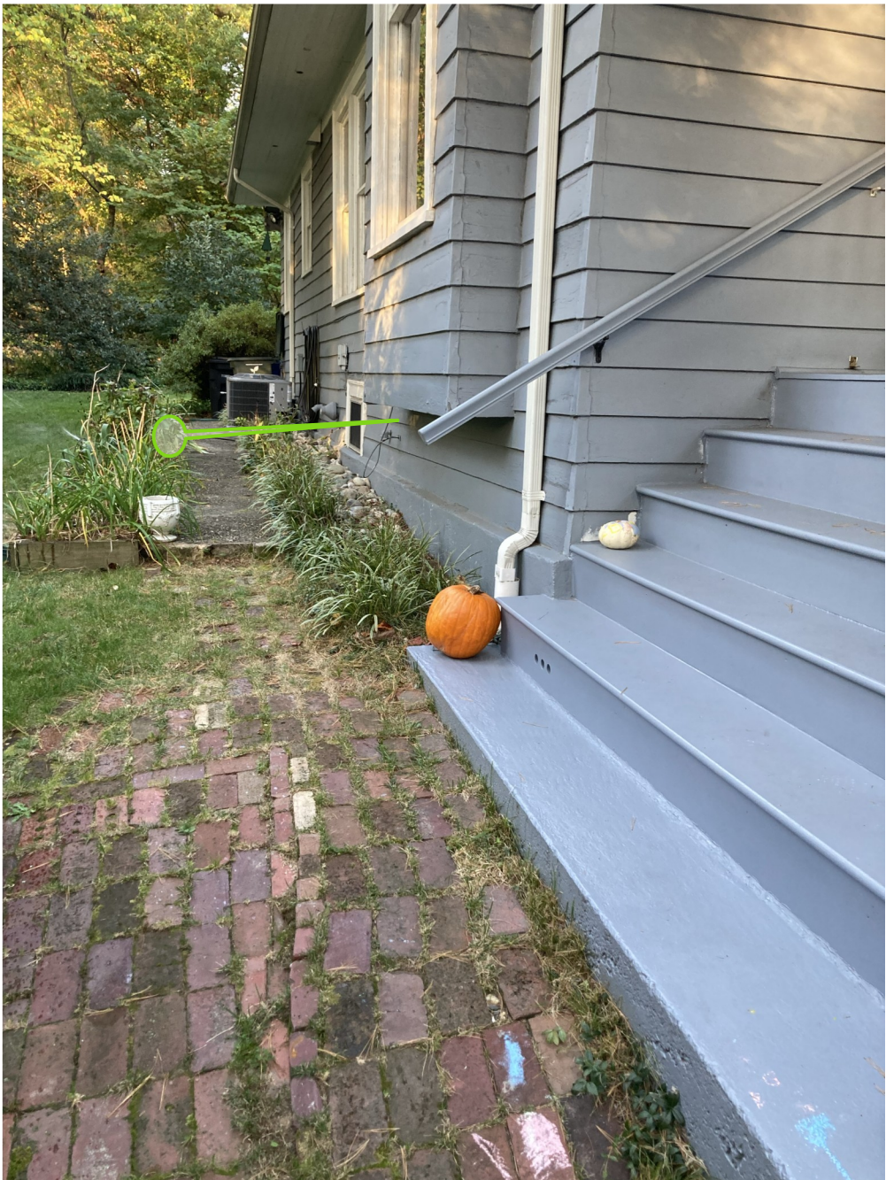
South side of residence taken from SE corner. Location of proposed charger on side of house near driveway.
