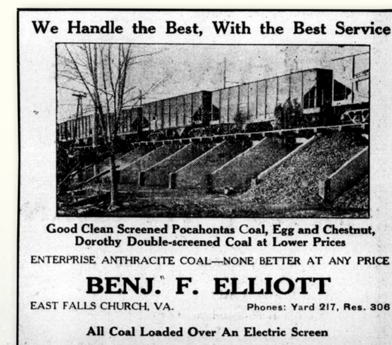
Above: Ad for Elliott Coal. Source: News-Observer, Nov. 17, 1927 Below: Coal trestle (center). Source: NOVA Parks / Photographed by Paul Dolkos.
