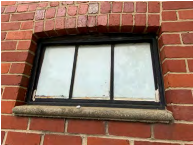
EXISTING BASEMENT WINDOW
