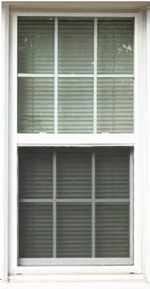
TYPICAL EXISTING WINDOWS (RETAINED)
