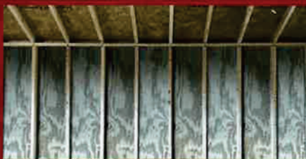
16" On-Center Studs & Trusses
