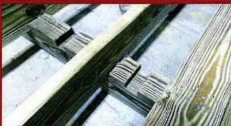
2x6 Pressure Treated Joists 2x4 are Standard
