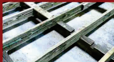
12" On-Center Floor Joists 16" OC is Standard
