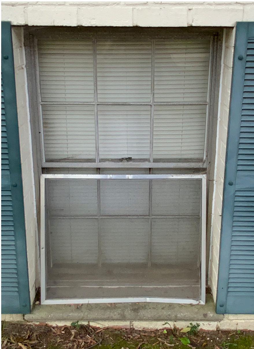
EXISTING ALUMINUM SASH WINDOWS
