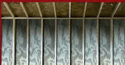
16" On-Center Studs & Trusses
