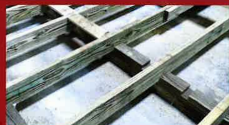
12" On-Center Floor Joists 16" OC is Standard
