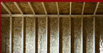
16" On-Center Roof Trusses
