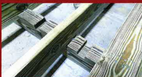
2x6 Pressure Treated Joists 2x4 are Standard
