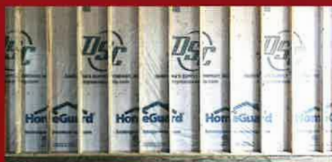
House Wrap Vapor Barrier Recommended if you plan to insulate
