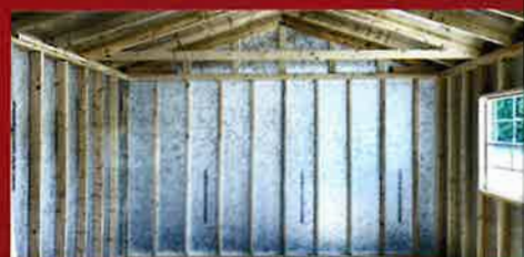
Tech Shield & Silver Tech Radiant Heat Barrier
