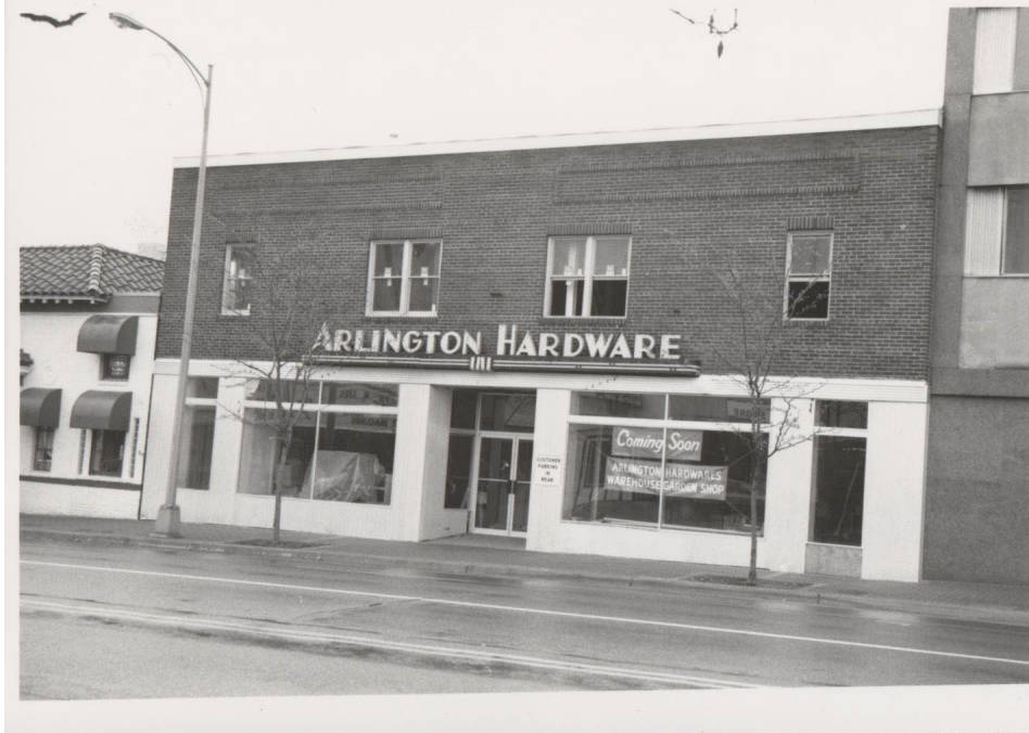
Figure 2: Photograph of the Arlington Hardware Building in April 1997 (Arlington County HPP)
