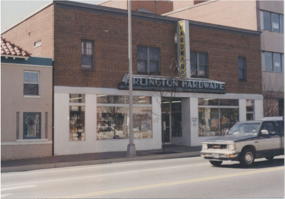
Figure 1: Photograph of the Arlington Hardware Building prior to the electrical fire in 1996 (Arlington County HPP)
