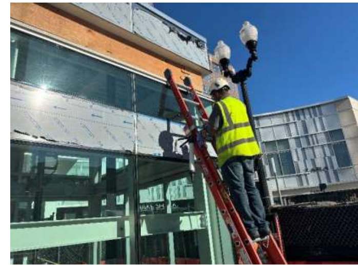
Applying caulk to glass at elevator headhouse
