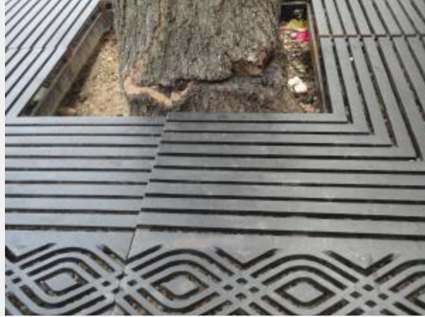
Trunk damage caused before grate was enlarged
