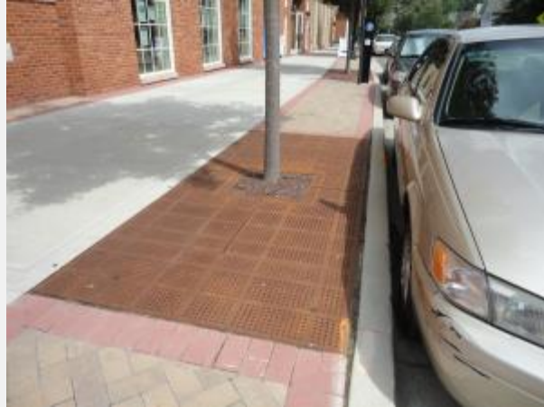
An example of a larger soil panel with sectioned grate that is easy to enlarge.
