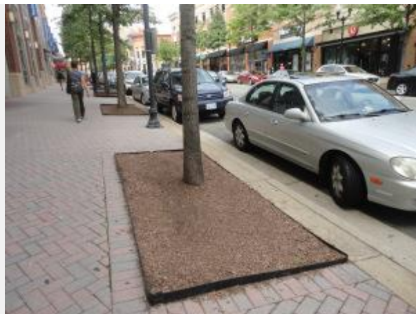
Larger spaces are provided for tree roots in the “soil panels” now required
