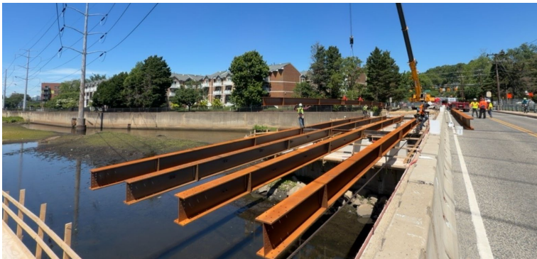
Arlington Ridge Road Bridge start ($19.1M)
