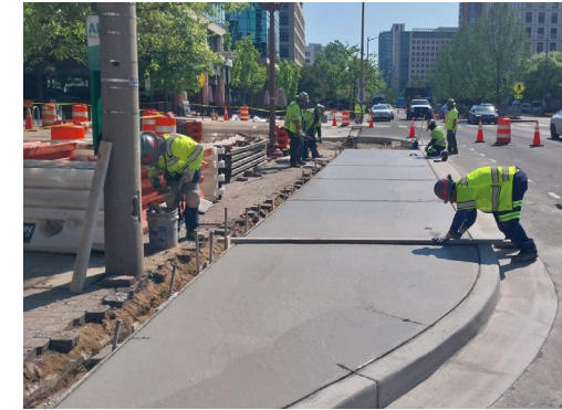
Countywide Spot Improvements: Fairfax Drive at North Utah Street
