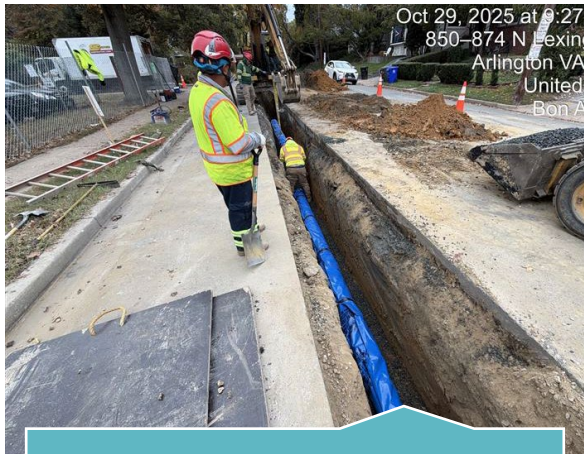
N Lexington St Water & Sewer Improvements
