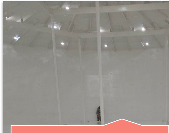
Fort Barnard Water Tank Rehabilitation
