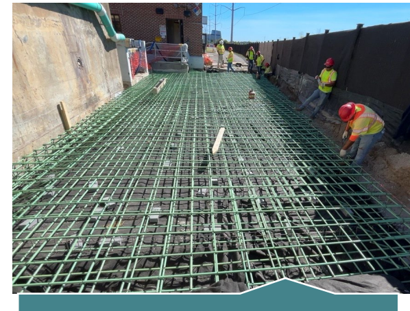
Sodium Hypochlorite Fill Station Rehabilitation
