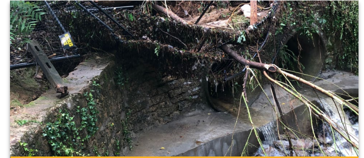
Military Road Culvert
