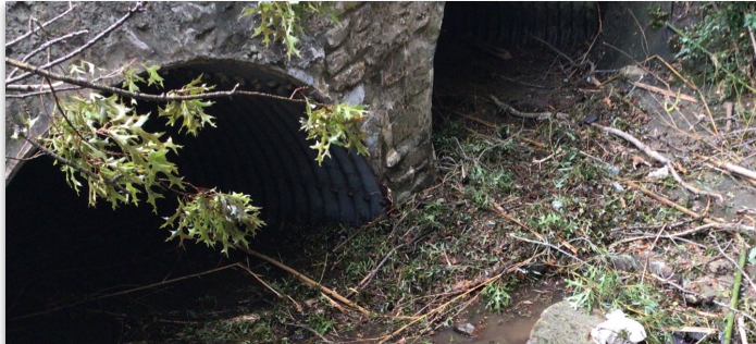
Dumbarton Culvert – Downstream
