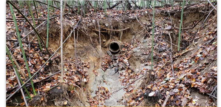
Gulf Branch Outfalls (Outfall Rehabilitation program)
