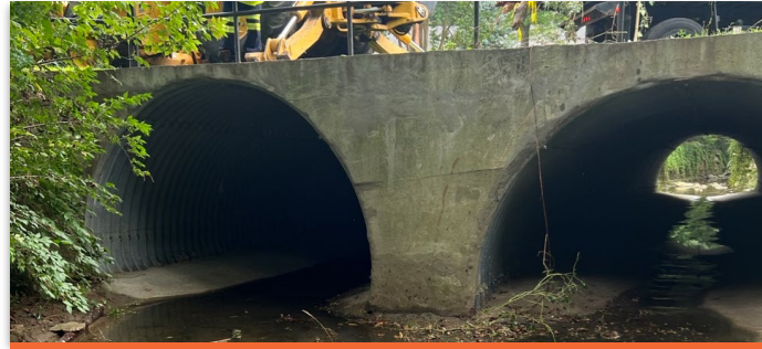
Dumbarton Culvert – Upstream
