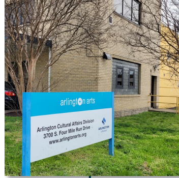
Cultural Affairs Boiler Electrification
