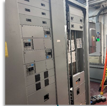
Court Square West Switchboard Replacement
