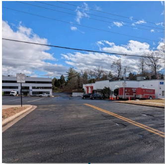
Quincy Site Access Control Gate
