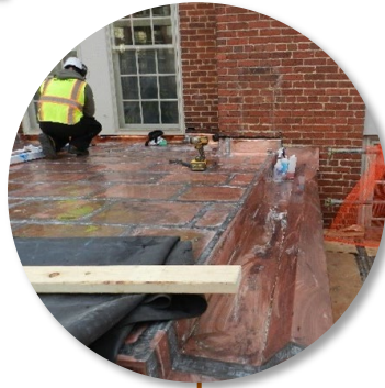
Museum of Contemporary Art Historic Portico and Roof Repairs
