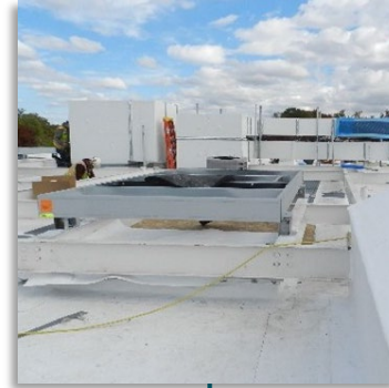
Quincy 2 HVAC Replacement
