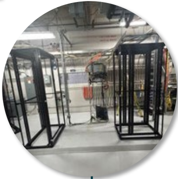
Bozman NOC Relocation to Detention Center
