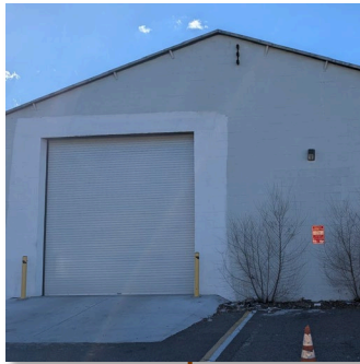
Oakland St. Warehouse Phase 2
