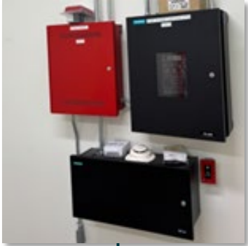
Fire Alarm Replacement - CSI
