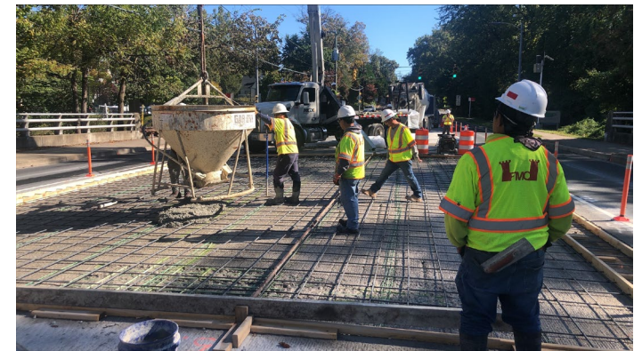
Wilson Blvd over Four Mile Run
