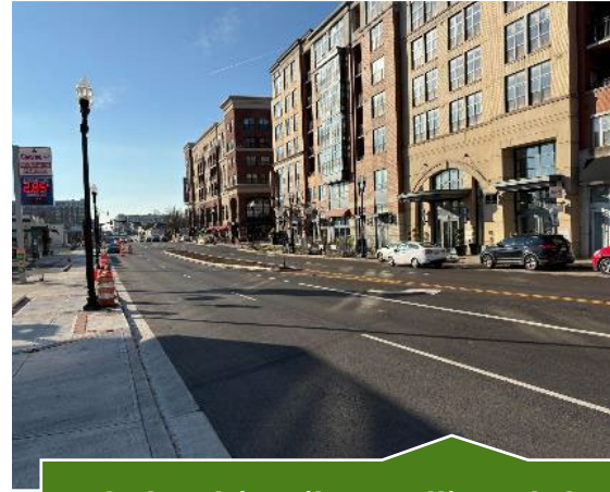
Columbia Pike Multimodal ($161M) Substantially Completed Dec 2025
