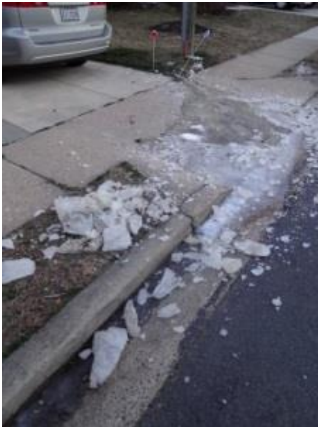
Ice from a sump pump discharging near a property line.
