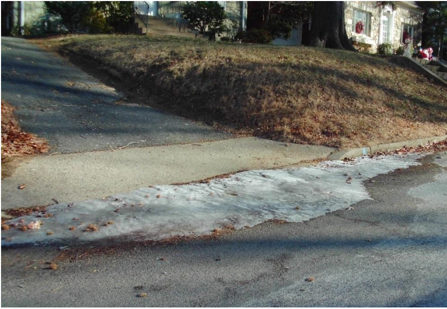
Accumulated ice in the gutter
