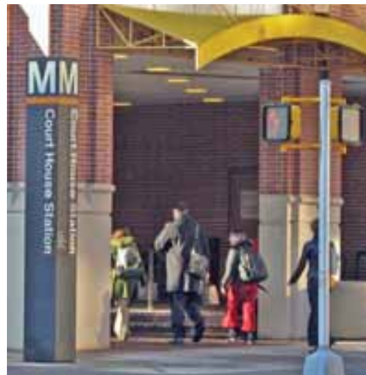
A Metro station in Arlington
