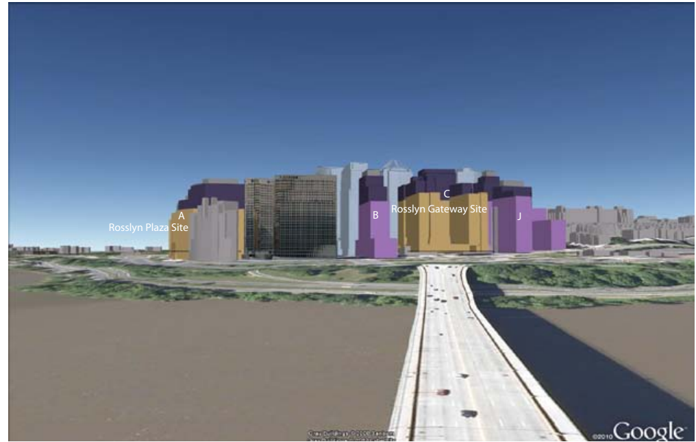
SKYLINE -- KEY BRIDGE LOOKING SOUTH
