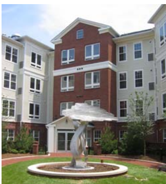
Sierra Condos, which began sales in 2005, include 10 affordable units.
