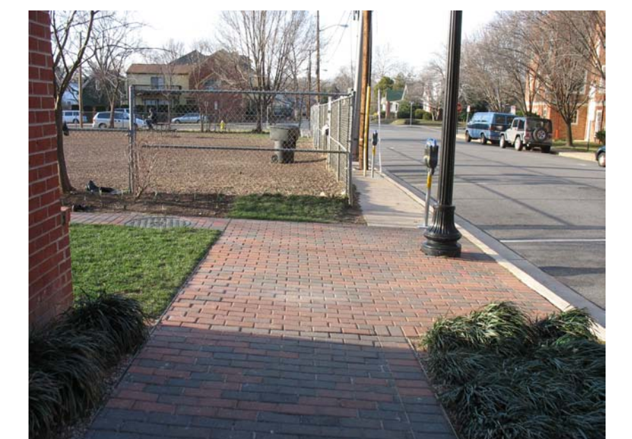
Wider Sidewalks On Hartford Street End At Existing Concrete Sidewalks At Park
