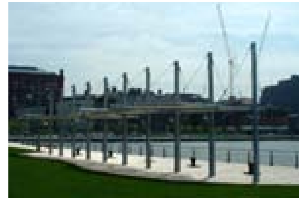
Structures In Hudson River Park NYC photos by fabric, inc.
