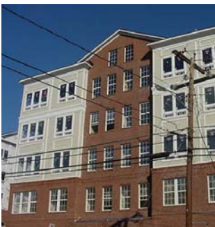
Sierra Condos shown under construction, include 10 affordable units.
