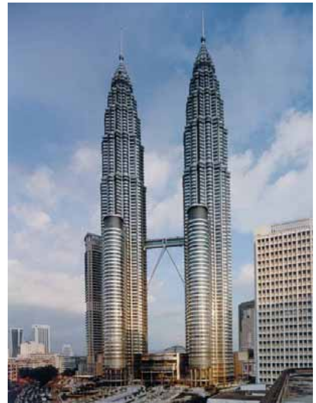
Petronas Tower Kuala Lumpur, Malaysia. Structural Engineer: Thornton Tomasetti Group MEP: Flack + Kurtz
